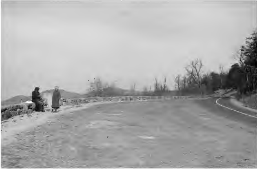
Skyline Drive (Virginia), 1937. The Skyline Drive in Virginia was the first rural parkway built by the federal government. Thousands of locals were displaced for the construction of the road. This image shows Hezekiah Lam and his daughter (described as “hollow folk”) waiting at a scenic stop for motorists to give them alms. Photograph by John Vachon, Library of Congress, Prints and Photographs Collection LC-USF33-001022-M2
