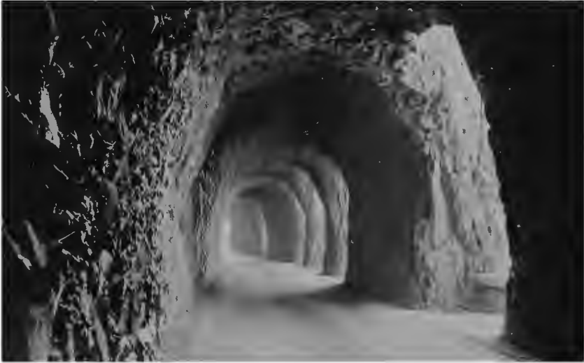
Mitchell Point Tunnel on the Columbia River Highway. Having toured Europe and its roads, road builder Samuel Lancaster emulated the Axenstrasse in Switzerland for some of the features of the Columbia River Highway in Oregon. The Mitchell Point Tunnel ( above ) aims to outdo its Swiss counterpart ( opposite ) by featuring five windows instead of three. Samuel Christopher Lancaster, The Columbia: America's Great Highway through the Cascade Mountains to the Sea , 3rd ed. (Portland, Oregon: J. K. Gill, 1926), 124
