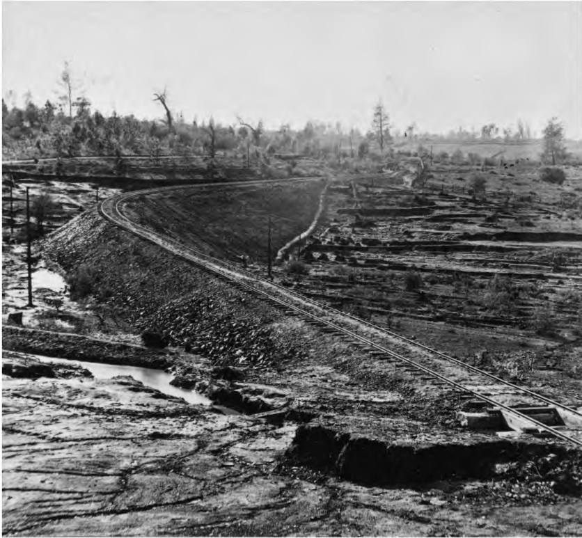
High embankment, near Auburn, California (1865). Railroad tracks impose a new geometry on the landscape and result in loss of timber. This image shows an embankment built for the Central Pacific Railroad in the foothills of the Sierra Nevada in California. Library of Congress, Prints and Photographs Collection LOT 11477, no. 11
